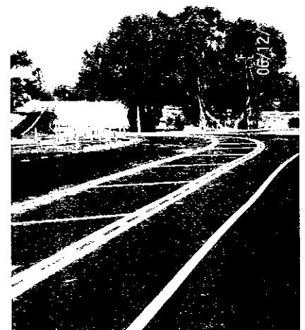
Coe Avenue intersection with General Jim Moore Boulevard — Phase III
